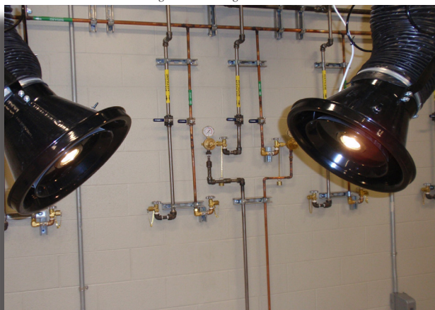
Welding stations and fume source capture arms.
