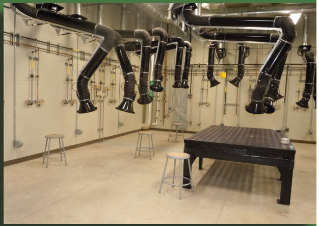
Sculpture room prior to placement of the student welding benches.
