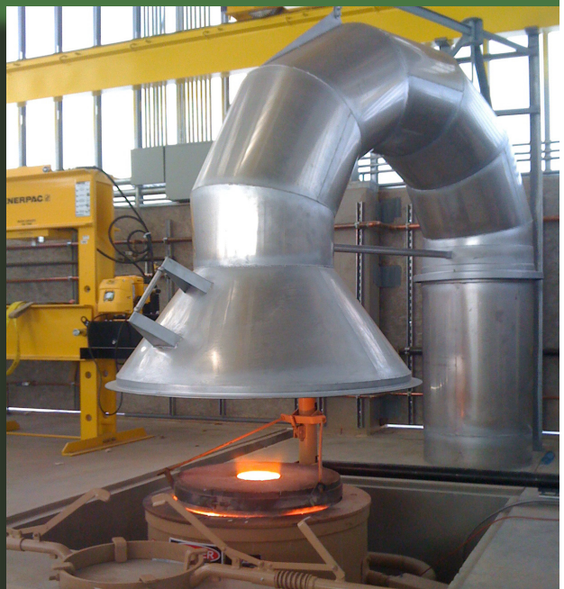
Finished condition of Foundry crucible and exhaust hood.
